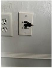
Courtroom 515 has podium hookups for the TV on the left wall of the courtroom. VGA and HDMI are available (An HDMI adapter to the VGA is connected at the podium). Both require the audio jack to be plugged in. The judge has control to turn audio on/off from the bench.
